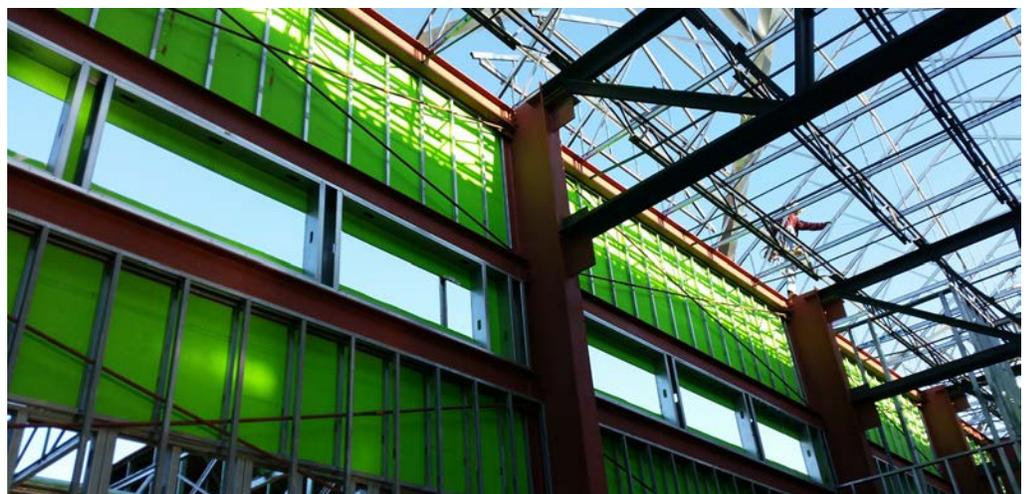
*The building design was that of a standard commercial building—gypsum sheathing panels over metal studs. Spray foam is excellent for this application because it adheres to the substrate and expands, creating a seamless air barrier. Also, spray foam will not buckle or sag, unlike traditional fiberglass batts, which commonly do.*
