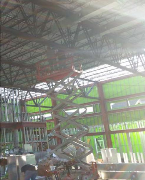
*Proper safety was a top priority on the job. When spraying the gymnasium area using a scissor lift, Profoam used straps and safety harnesses at all times.*
