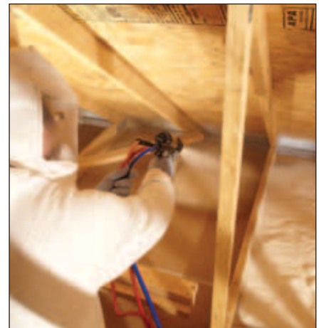
Spray - Ideal for attics and rim joists.
